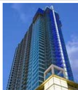
The Spire soars into the sky and condos in the tower are doing the same. (Photos courtesy of Frank Ooms.)
